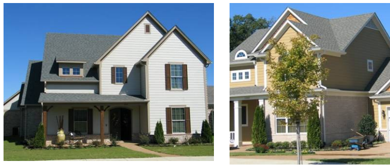
These two VESTA 2009 homes, built by Jon Ruch Builders (left) and Regency Homes (right) not only met EcoBUILD and NAHB program requirements, but also attained NABH's Silver rating for added green features.
