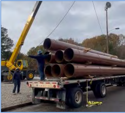
Weaver-Gill pipeline project.
