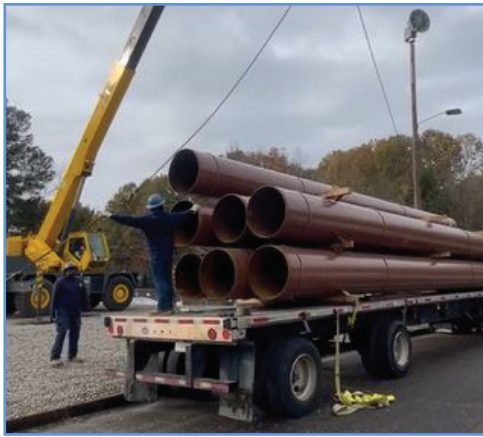
Weaver-Gill pipeline project.
