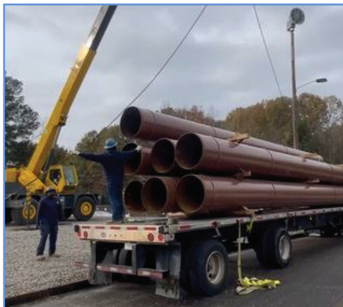
Weaver-Gill pipeline project.
