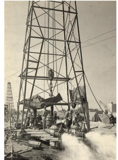
This historical photo from the early 1930's shows a new well at Sheahan Pumping Station that is being tested to see how many gallons are being produced per minute to verify that it is at the correct productivity level rating.
