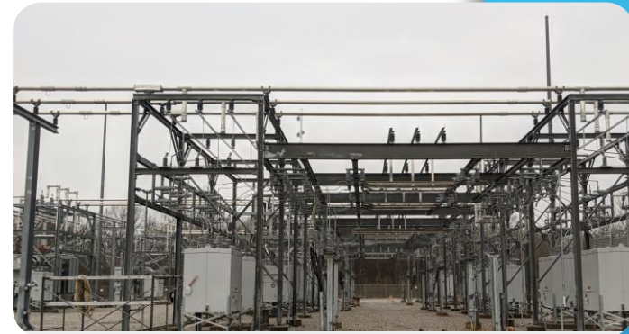
New electric substation 89
