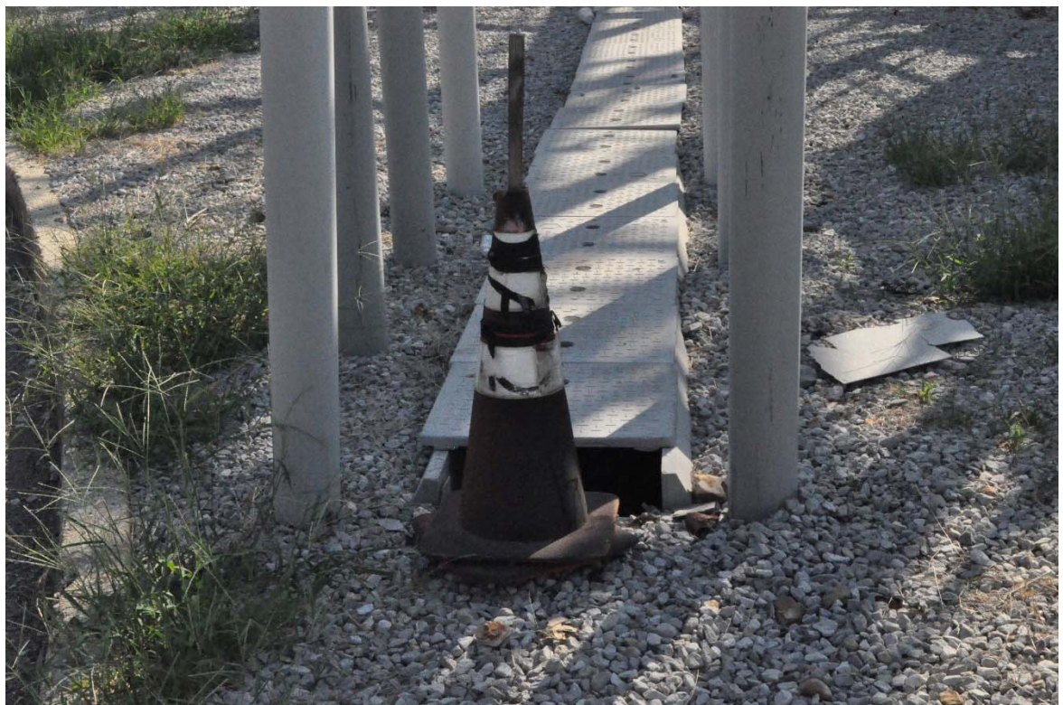
Figure 3-13. Substation #3 – cable trench issue
