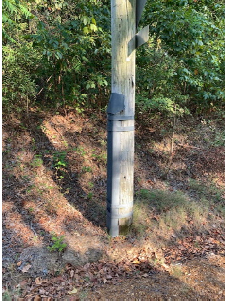
Figure 3-14. Steel truss/stub
