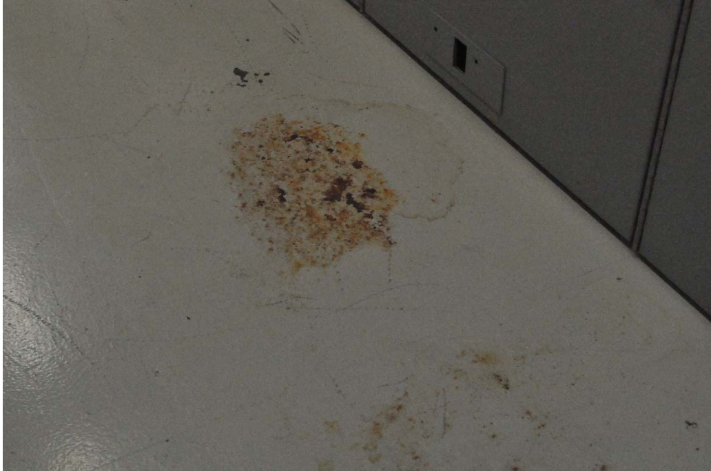
Figure 3-10. Substation #76 – Rust from water incursion inside the switchgear building
