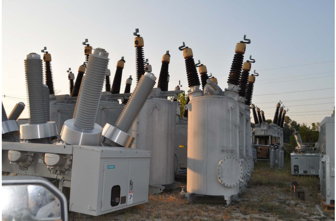
Figure 3-7. Spare breakers sitting inside the substation fence at Station #33
