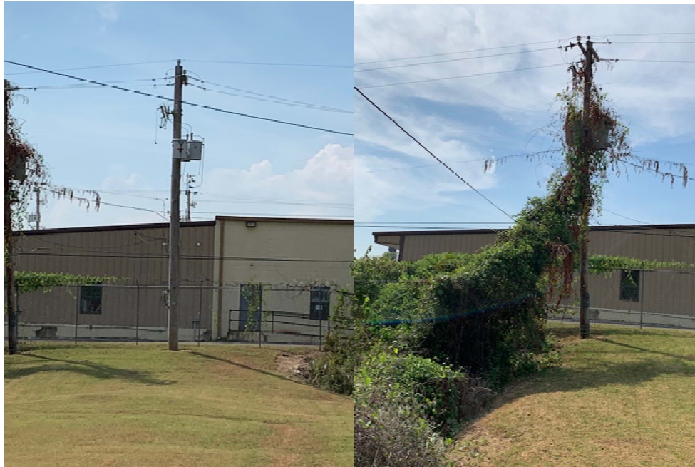
Figure 3-6. Examples of unused transformers
