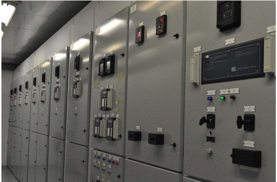
Figure 3-12. Substation #3 Switchgear Line-up
