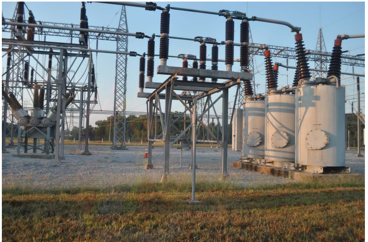
Figure 3-8. Main Bus Tie breaker at Station #33.
