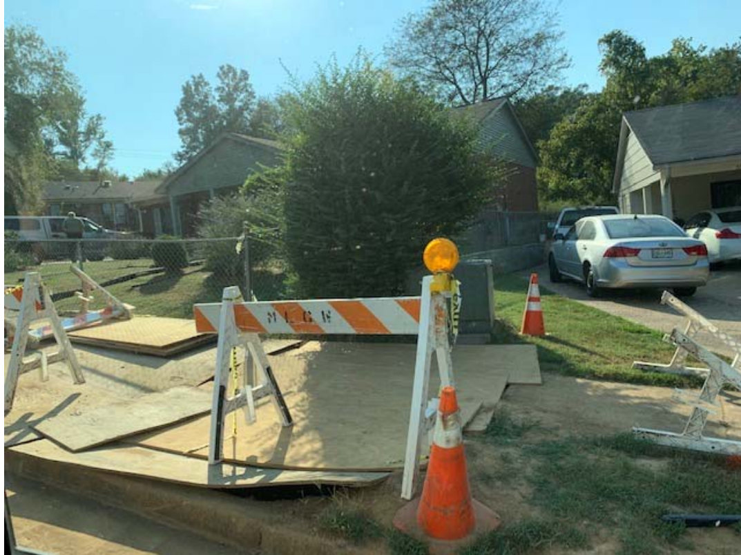
Figure 3-155. Unfinished underground cable project
