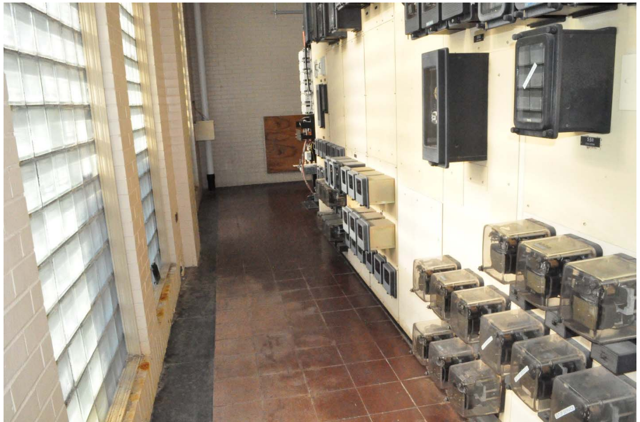
Figure 3-11. Substation #5 – Relay Panel Line-up
