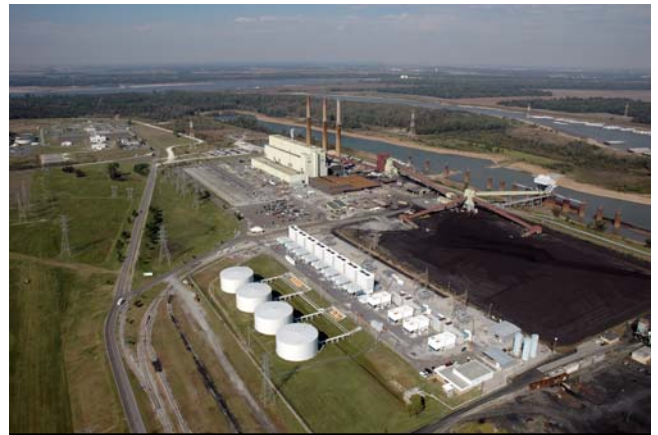
An aerial view of TVA's Allen Fossil Plant located in southwest Memphis.
