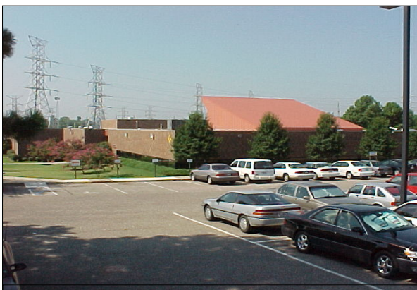
MLGW's Joyce M. Blackmon Training Facility proved a cost-effective location to deploy occupancy sensors. The energy management project is expected to have a one-year payback.
