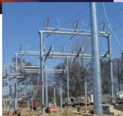
Construction began in 2004 on this substation, which will provide added reliability to the St. Jude and Uptown area of downtown.
