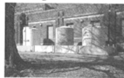
The 2008 budget will provide for seismic improvements to Sheahan water pumping station.
