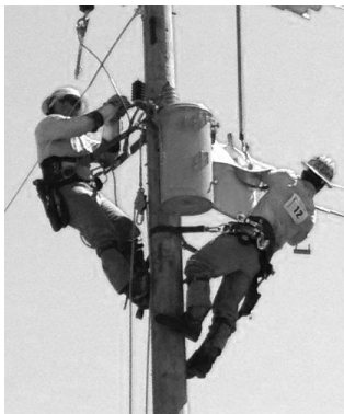
Huston and Smith compete in the blown transformer event.
